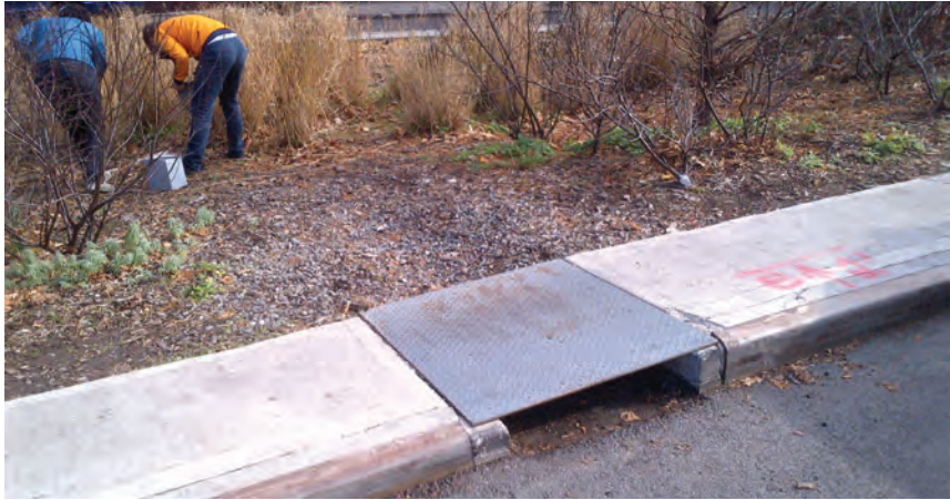
ABOVE: Enhanced tree pit detail in the Bronx showing the stormwater inlet
