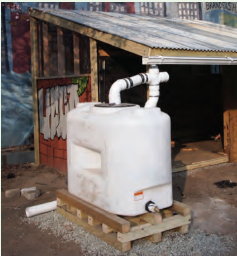
ABOVE: Rain water harvesting structure in a Manhattan school garden
