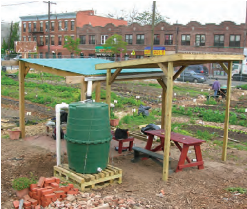
Rain water harvesting setup
