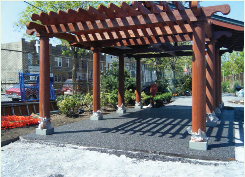
ABOVE: Permeable paving installed under an arbor at a community garden in Brooklyn
